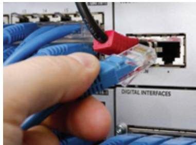
Data Cabling Installations and Relocations
